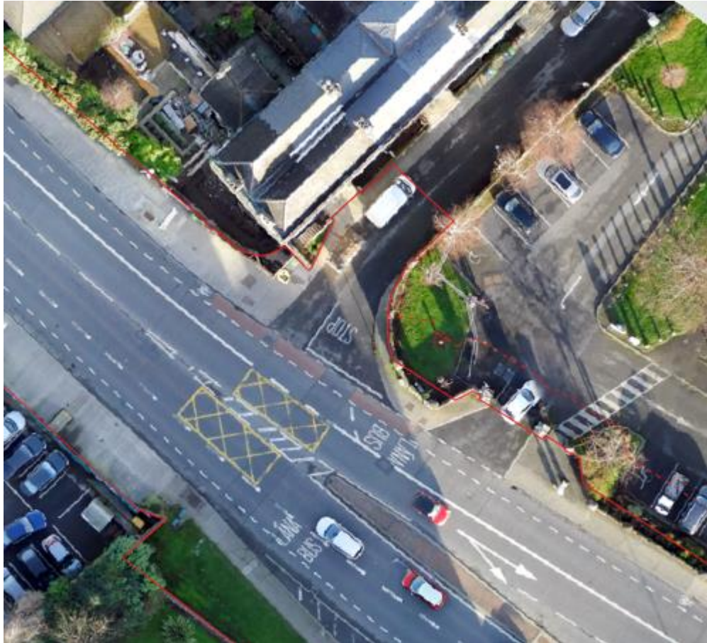
Figure 4.1: Extent of land take at the corner of Phoenix Terrace / Blackrock Park (Image Source: Google)
