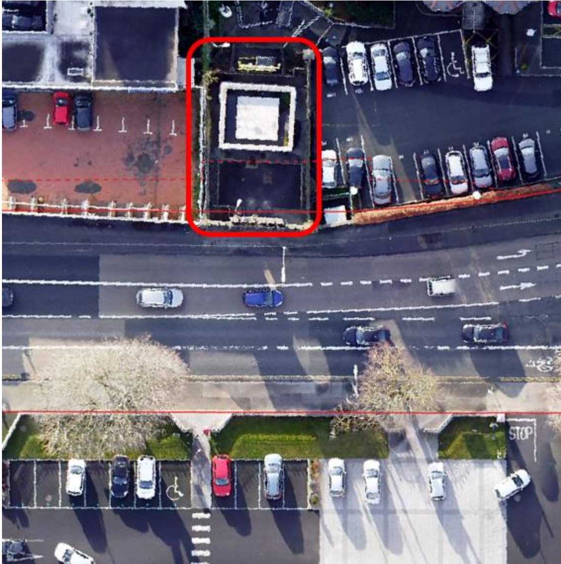
Figure 3.54: Existing aerial view at St. Vincent's AGI (Image Source: Google)
