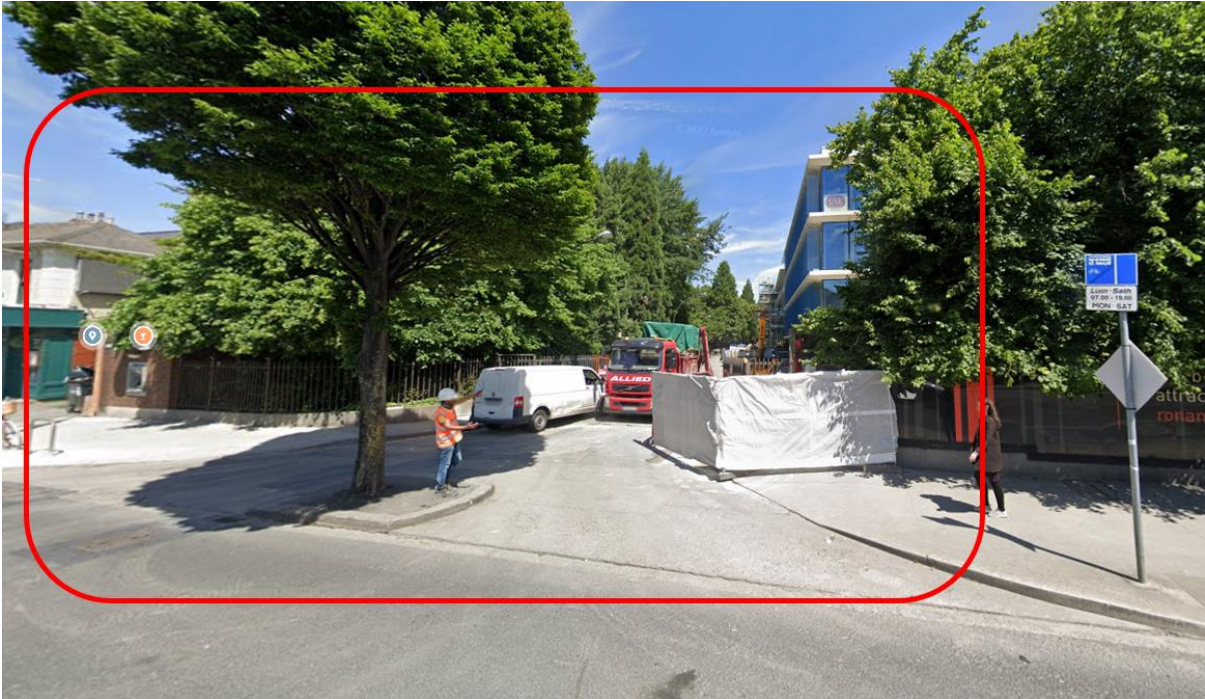
Figure 3.11: Existing Street View of Meta, Merrion Road (Image Source: Google)
