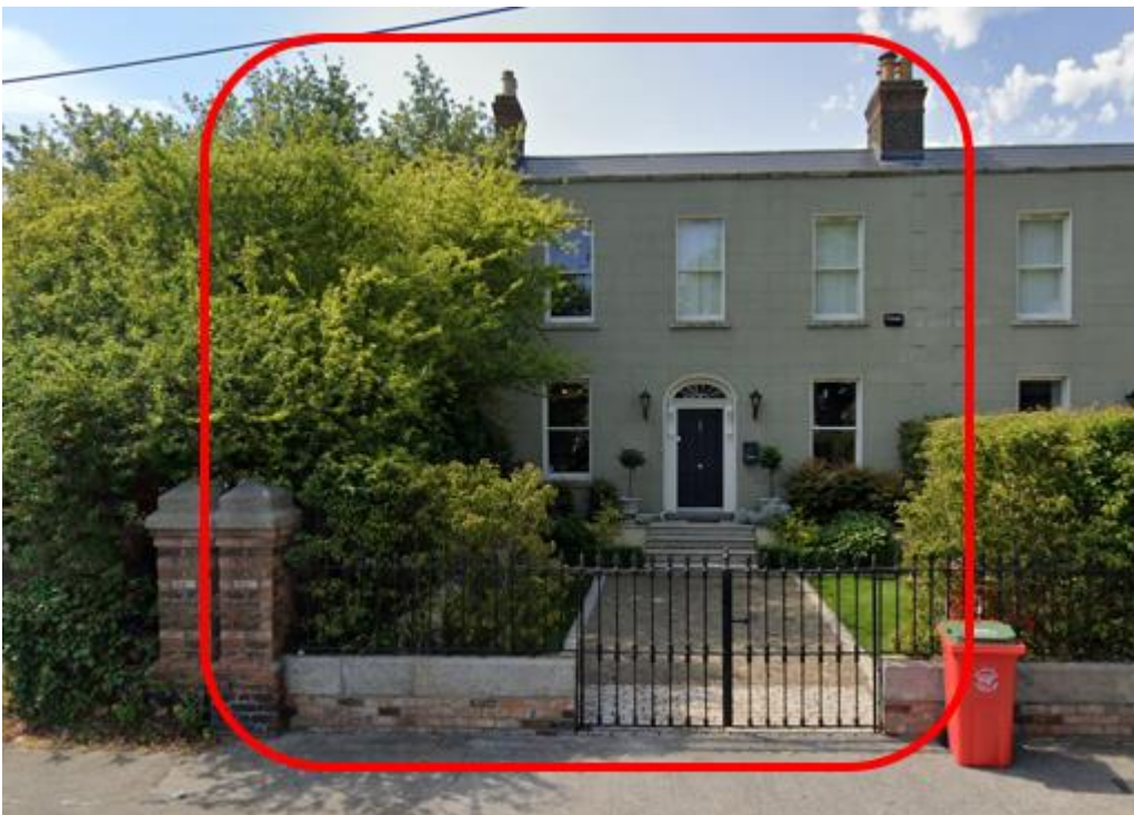
Figure 3.75: Existing Street View at (Image Source: Google)
